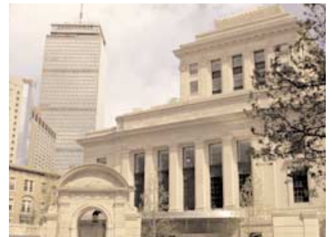
The new front of The Mary Baker Eddy Library.
