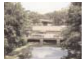
A section of the Charlesgate Dredging Project.
